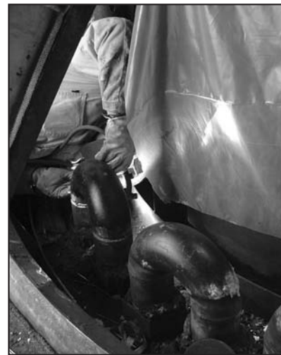
A Turnaround Welding team member performs welding returns on a heater.
