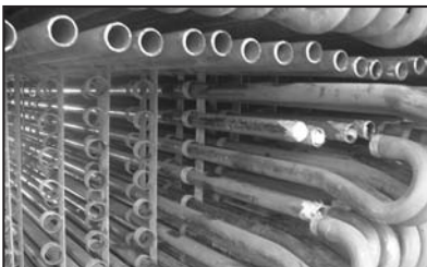
Retubing of an economizer completed by Turnaround Welding Services.
