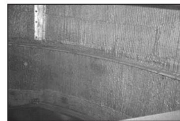
A weld overlay inside a reactor performed by Turnaround Welding Services.
